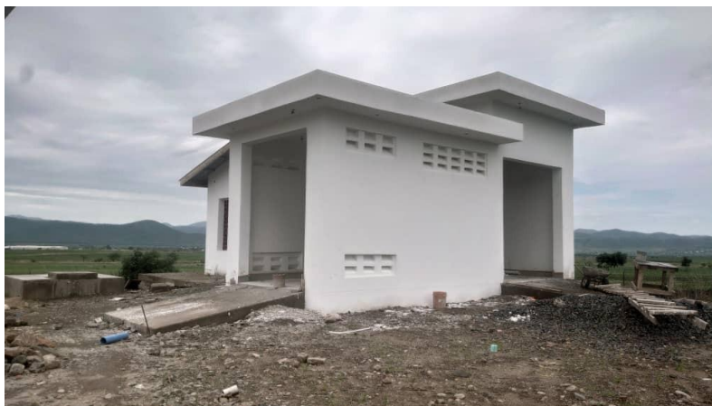
Photo 6: Upper air Station building at Songwe airport - December 2025
