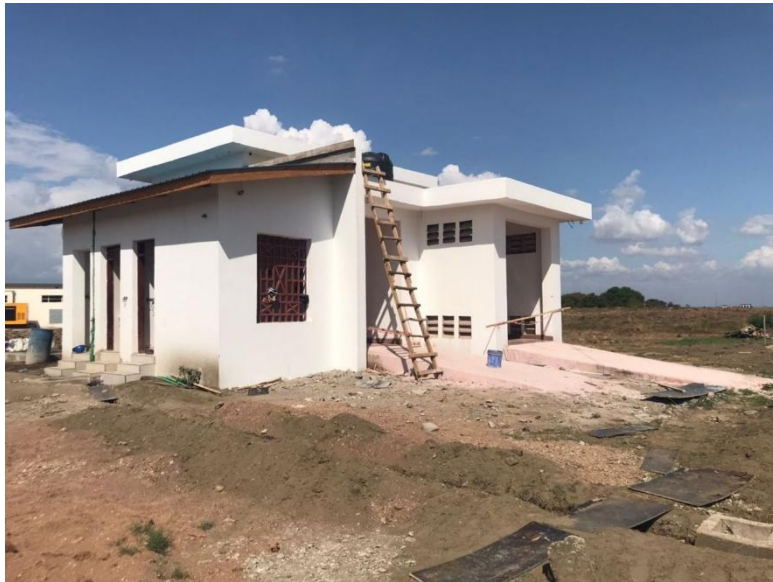
Photo 5: Upper air Station building at Kilimanjaro International airport - December 2025
