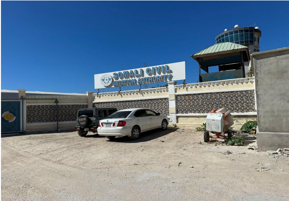
SCAA Office Complex at Mogadishu Airport
