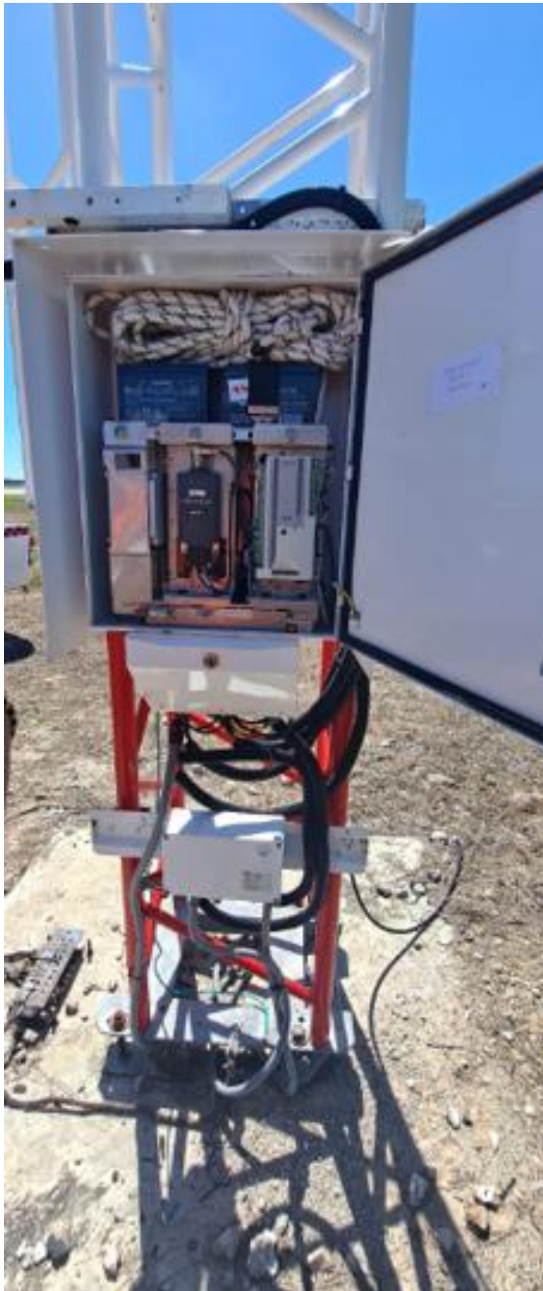
Figure AI.3. IDAC (Dominican Institute of Civil Aviation) automatic weather station at RWY 26 of the Punta Cana airport.
