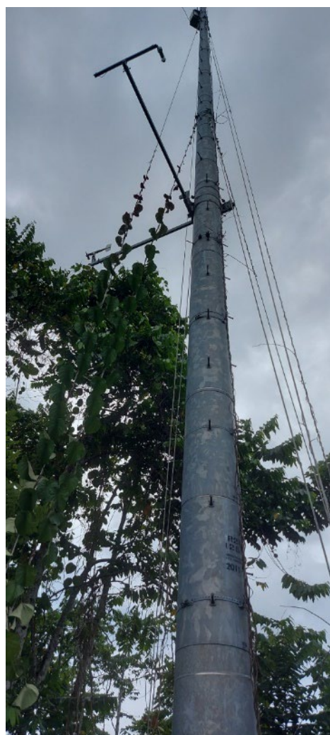
Figure 6. AWS at Maota Airport site showing climbing pegs and encroaching vegetation
